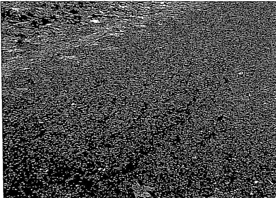
T470 - Valley Drive View of Fatigue Cracking
